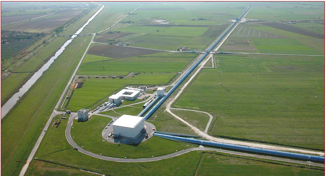
FIGURE 1.11 Aerial view of the Virgo interferometer near Pisa, Italy, showing the Mode Cleaner, the main building, the 3-km western arm and the beginning of the northern arm. Source: The Virgo Collaboration, Wikimedia Commons.
