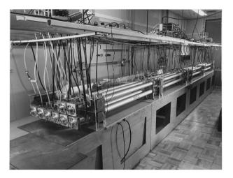
**Fig. 14** To generate 1.5 kW in the late 1960s, Hughes Research Laboratories passed the output of a 10-m  $CO_2$  oscillator through a 12-m preamplifier and a 42-m amplifier. The tubes were folded to fit onto a 32-×4-ft plywood table. (Courtesy W. Bridges)
