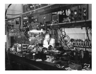
Fig. 5 Alan White working behind the optical bench holding the first red helium-neon laser at Bell Labs. (Courtesy of Alan White)
