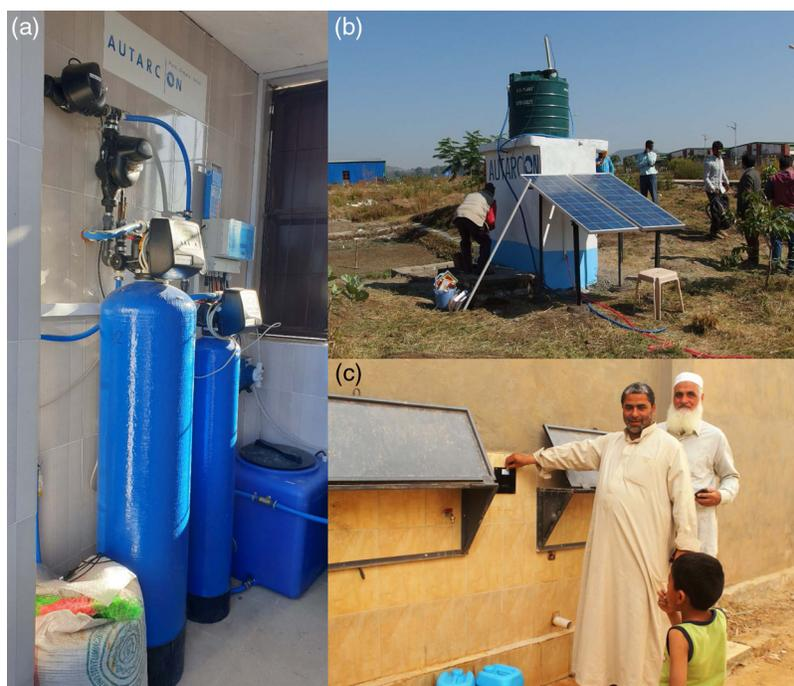
**Fig. 1** Autonomous PV powered system for cleaning and disinfection of drinking water based on anodic oxidation and *in situ* production of chlorine by an inline-electrolytic cell. Autarcon system installed in a rural setting. Water tapping with prepaid cards. (a)–(c) Photos courtesy of Philipp Otter, Tina Jaskolski.
