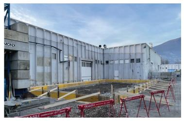
Figure 2. Concrete diaphragms, 13.5 m deep, define the rectangular well
